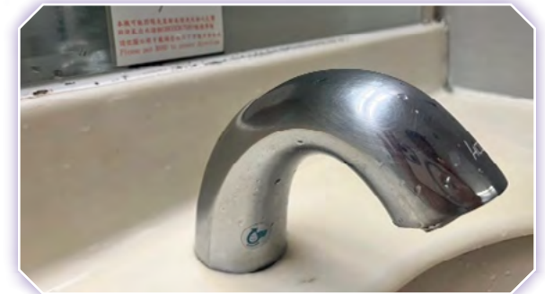
Adoption of sensor faucets with water-saving labels
