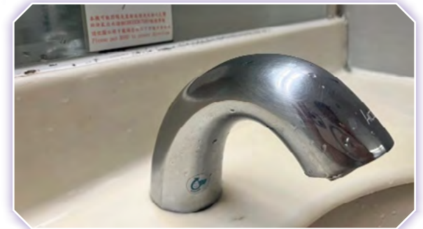
Adoption of sensor faucets with water-saving labels
